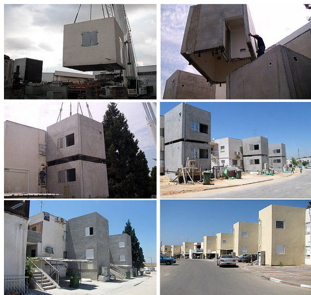
Figure 1. Fortified room Mamad during and after construction
