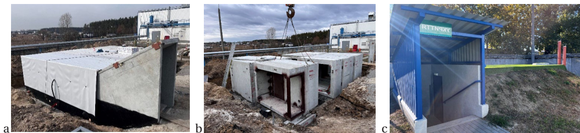
Figure 4. The simplest type of precast reinforced concrete shelter built at a factory in the Kyiv region
