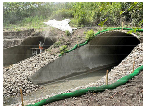
Figure 1. A practical example of the restoration of a corrosion-damaged corrugated metal pipe using GeoSpray geopolymer coating
